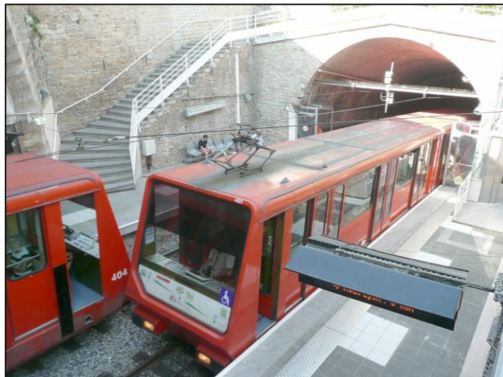
Trains on the St Just funicular passing at the Théâtres Romains station.
